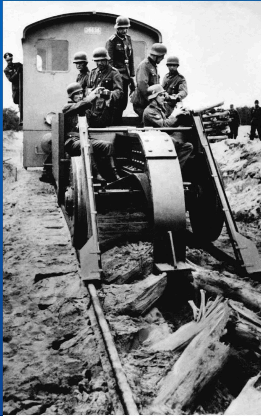
Schienenwolf destroying rail tracks during German retreat, 1944.
