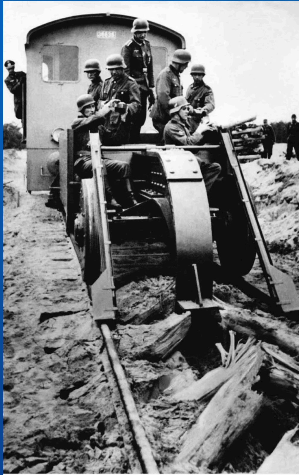
Schienenwolf destroying rail tracks during German retreat, 1944.
