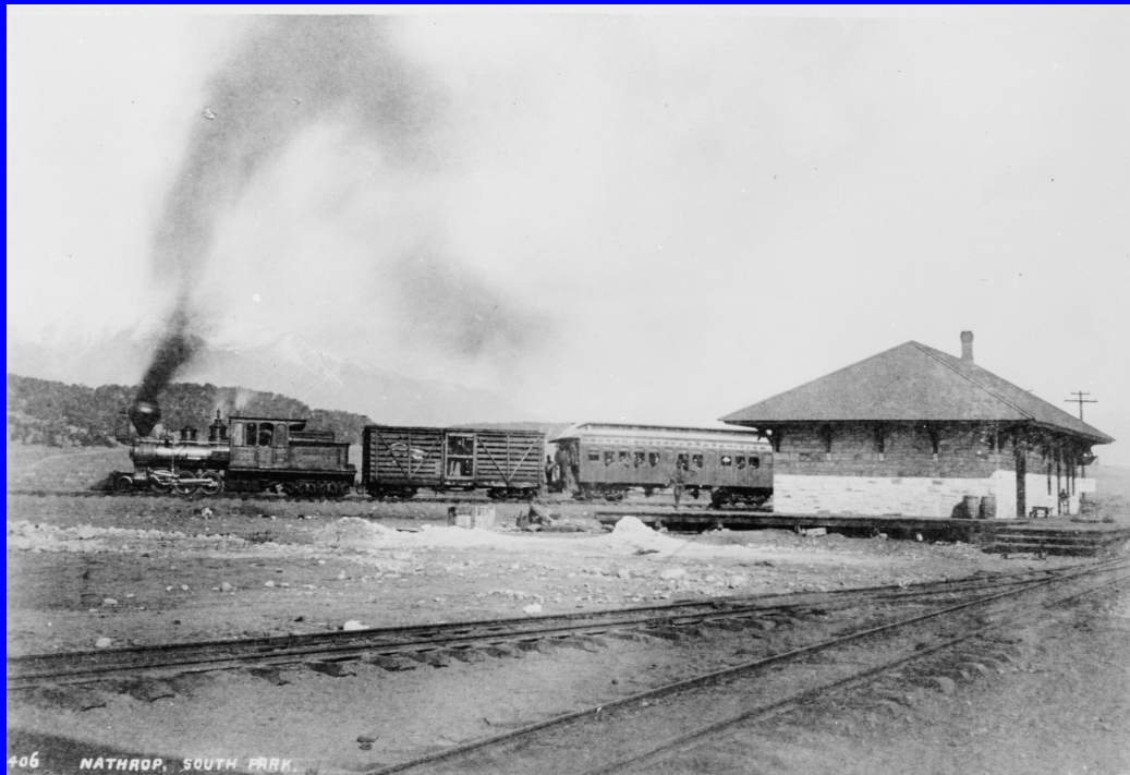
Mason-Bogie with DSP&P mixed train at Nathrop Depot interchange with D&RG
