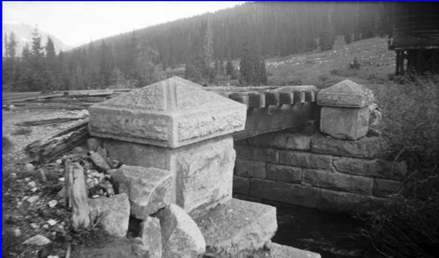
DSP&P bridge at Hancock, east of Alpine Tunnel
