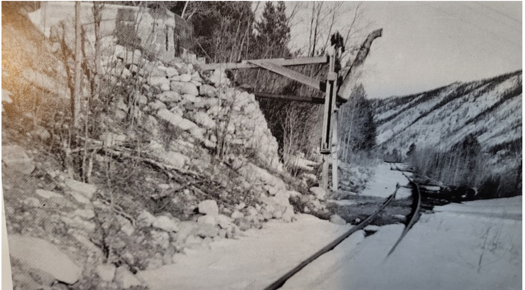
Garfield Water Column, gravity fed from a concrete cistern above the grade, located above the Monarch lodge.
