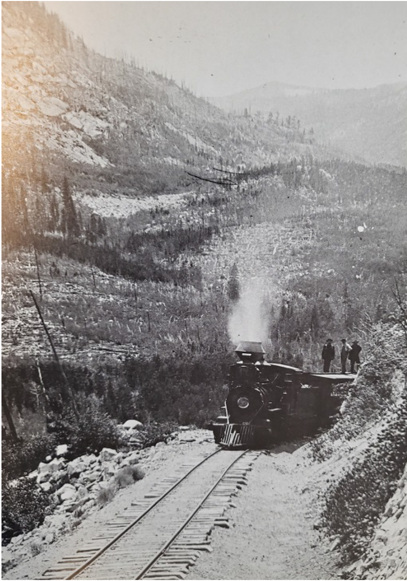
1880s, original rough cut ties, middle leg of Switchback
