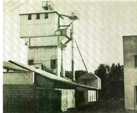
Concrete plant, another Raeford industry serviced by A&R, is notable for its tall mixing tower.
