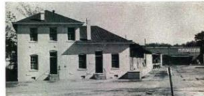
Side view shows terminal trackage at the station.
