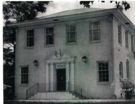
From the front, Fayetteville station is another stately structure in the A&R tradition.
